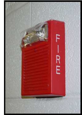
Fire Alarm Horn/Strobe
